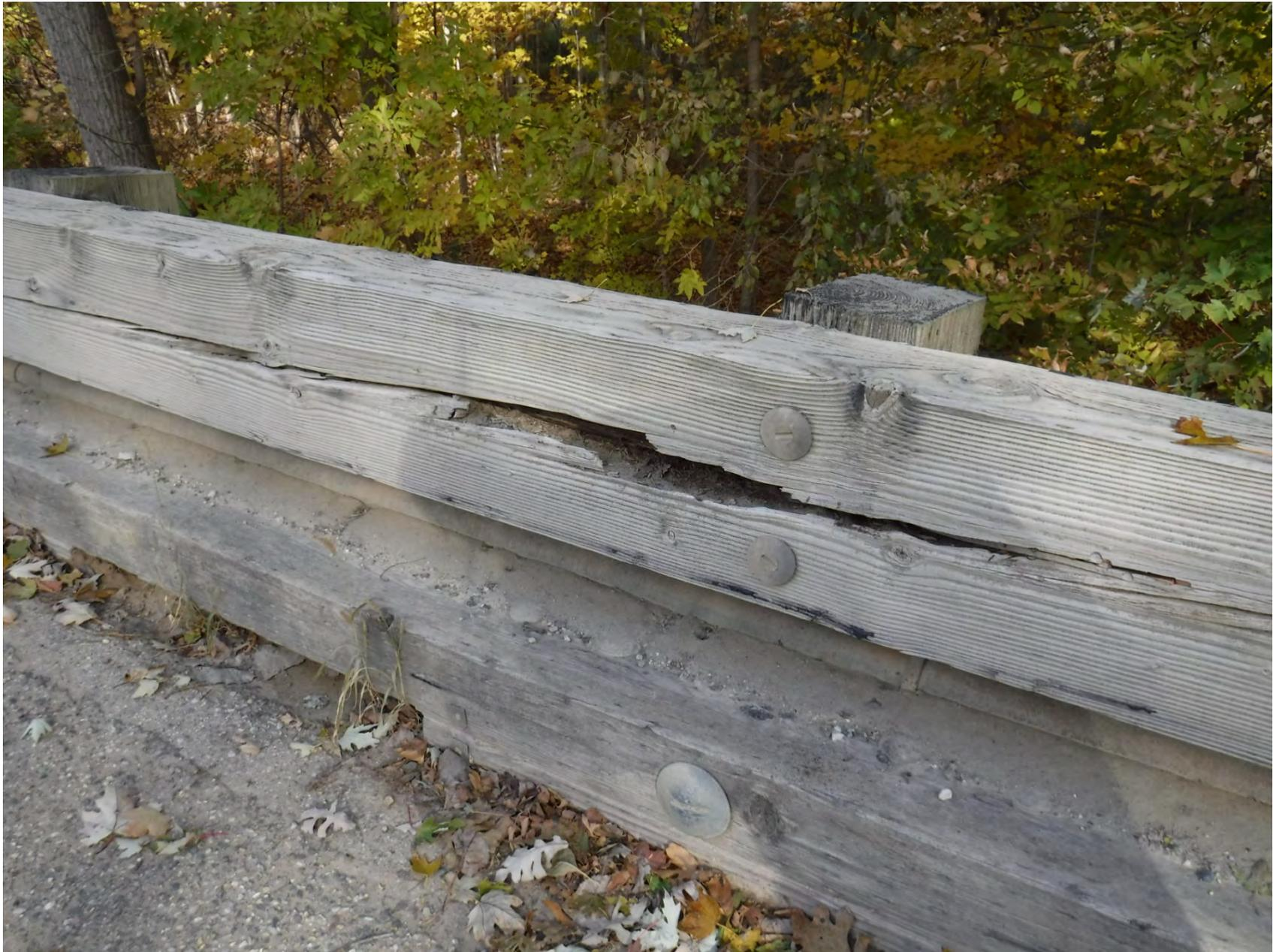
ROTTING AREA ON NORTH RAILING IN SPAN 2W
