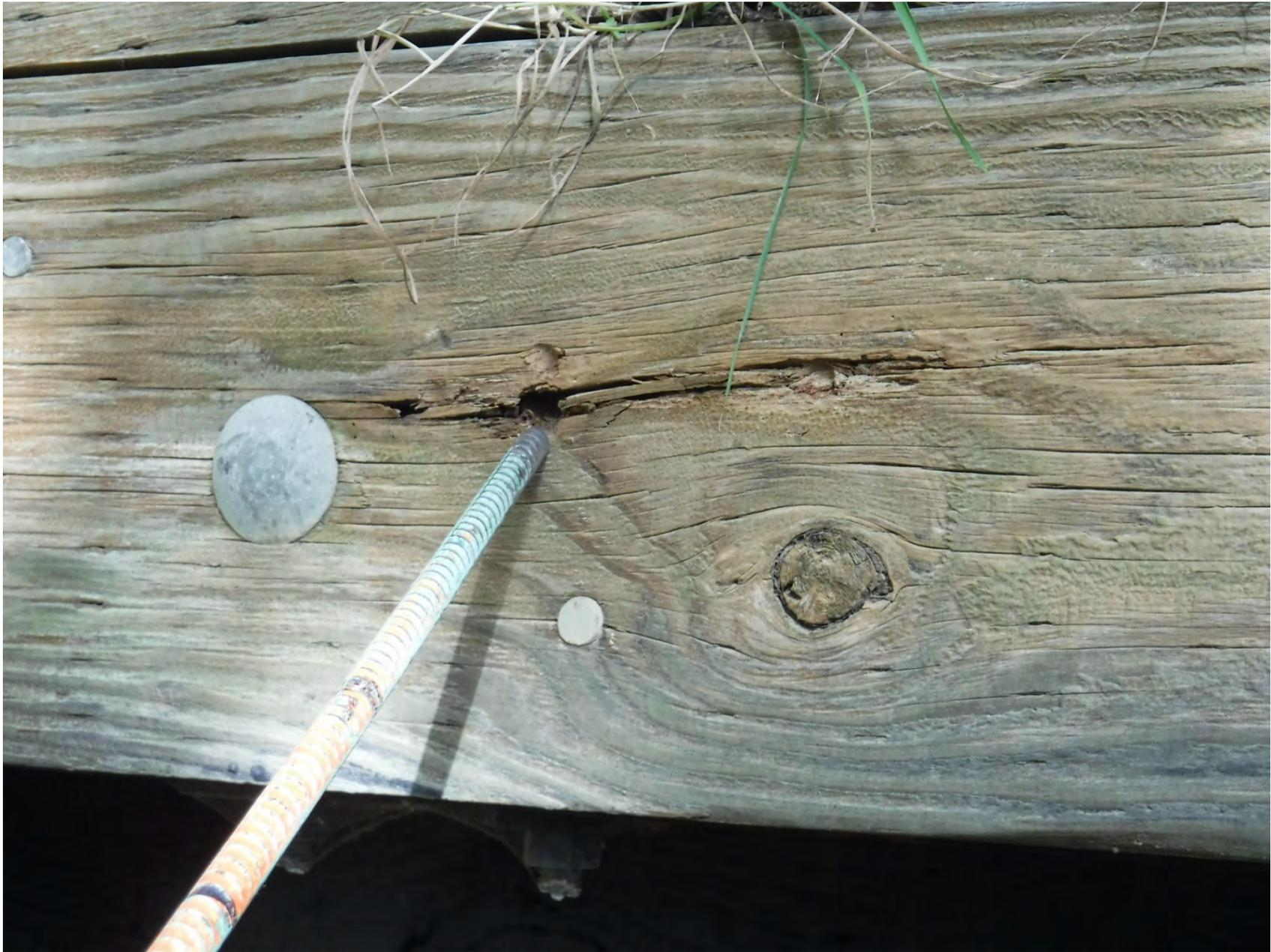
ROT STARTING IN SOUTH FASCIA NEAR MIDDLE OF SPAN 1E
