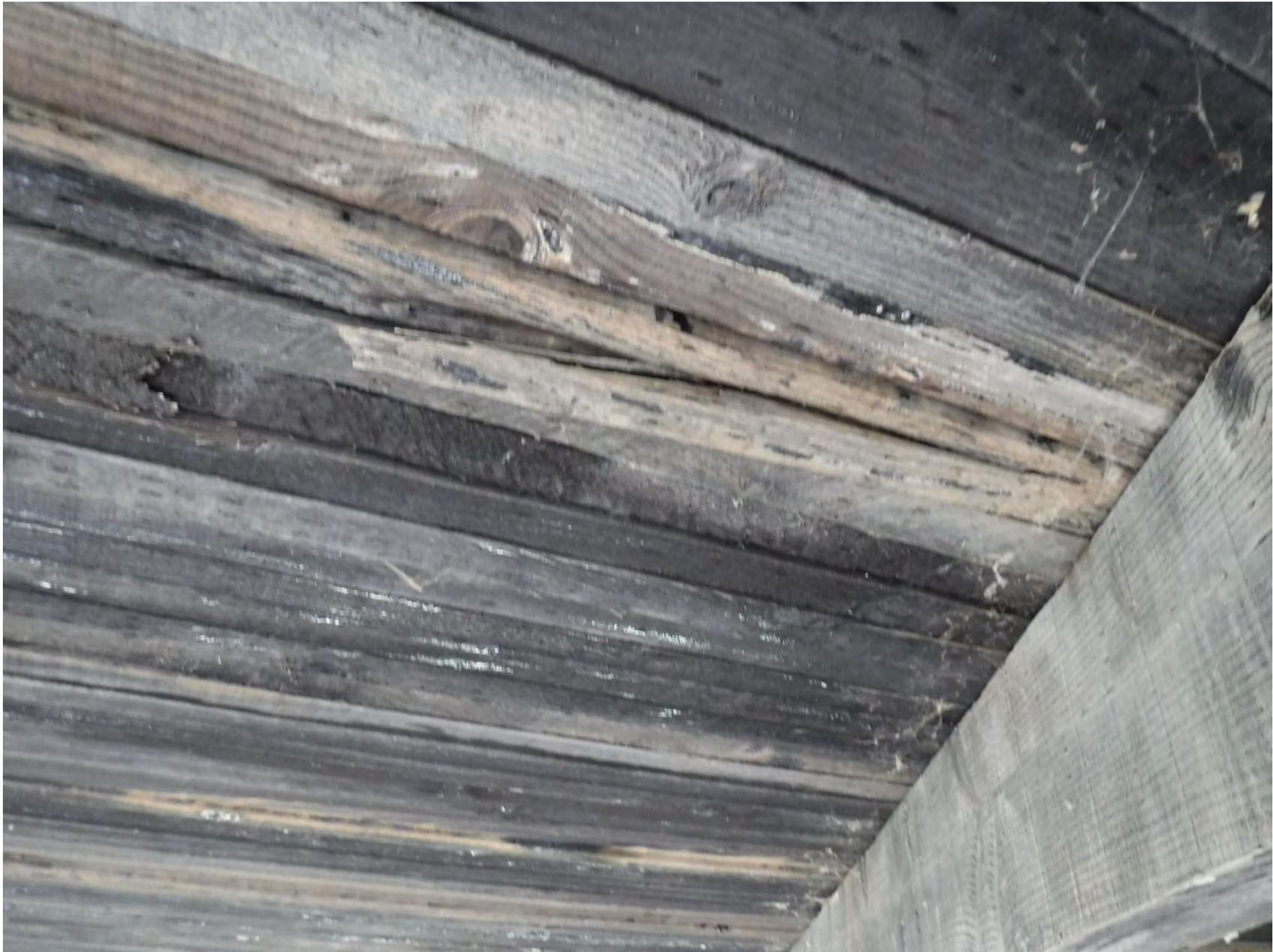
BROKEN DECK BOARD IN SPAN 1E WEST OF SPREADER
