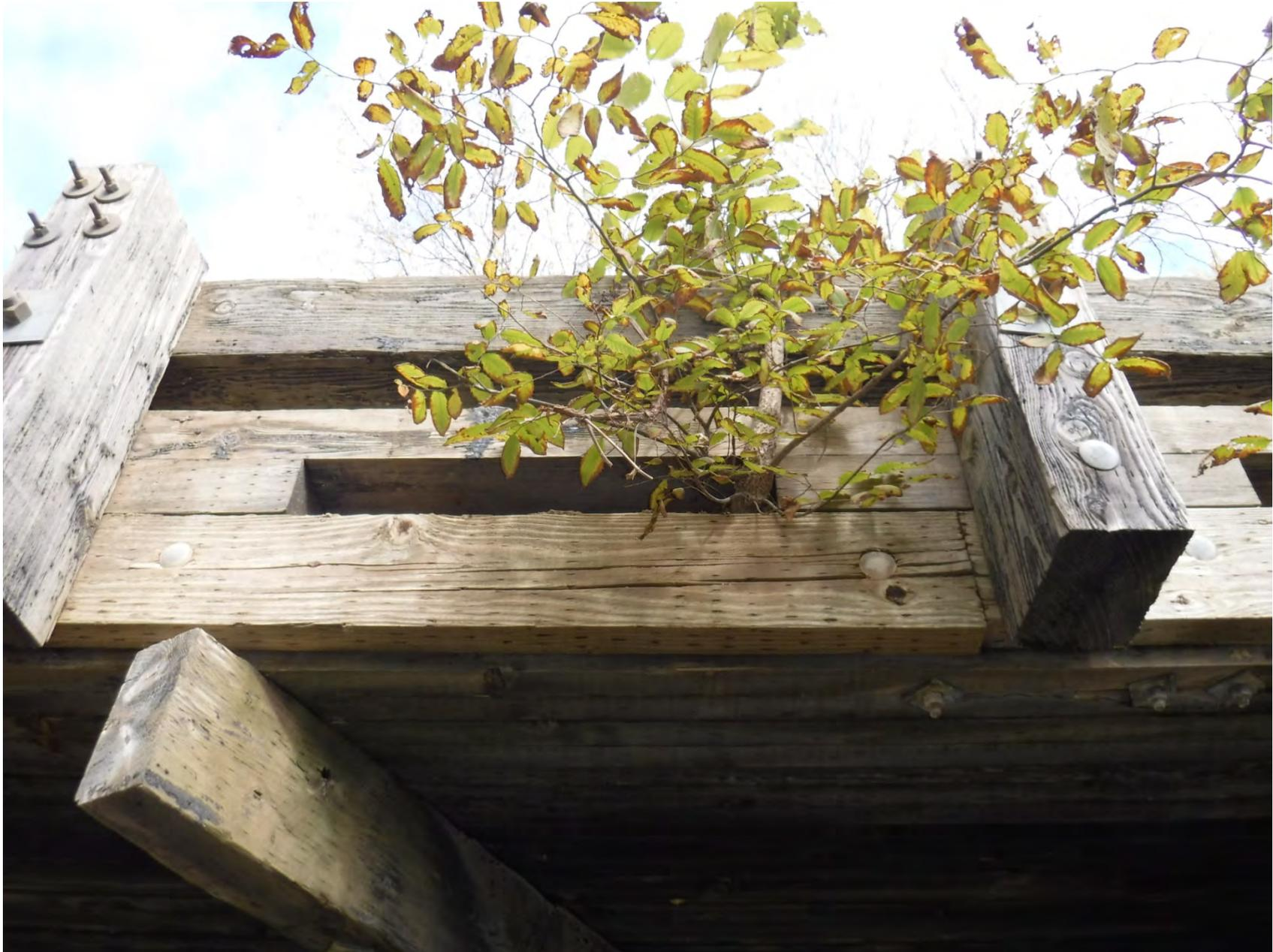
CHECKING IN SOUTH FASCIA NEAR MIDDLE OF SPAN 1W
