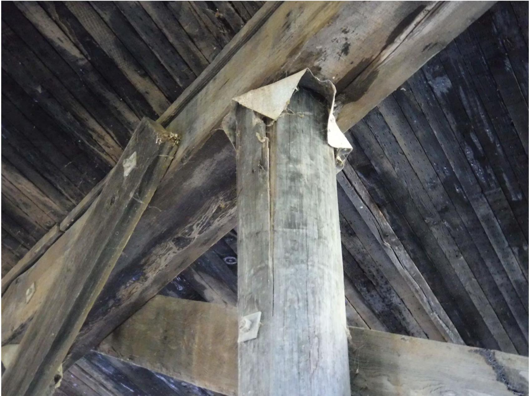
SPLIT IN EAST FACE OF PILE 3N IN PIER 2E
