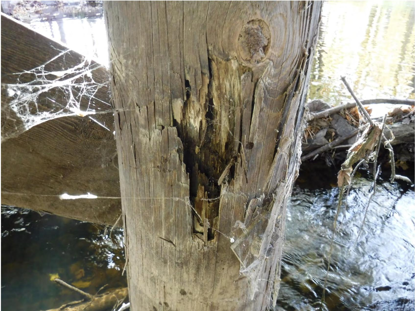
ROT STARTING ON PILE 3S IN PIER 3E
