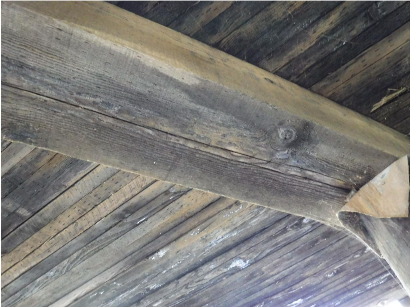
CHECKING ALONG BOTTOM OF PIER 1E CAP
