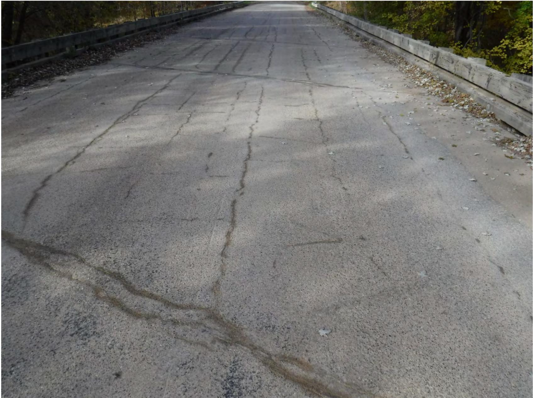
LONGITUDINAL CRACKS IN HMA SURFACE OVER BRIDGE WITH MAP CRACKS DEVELOPING
