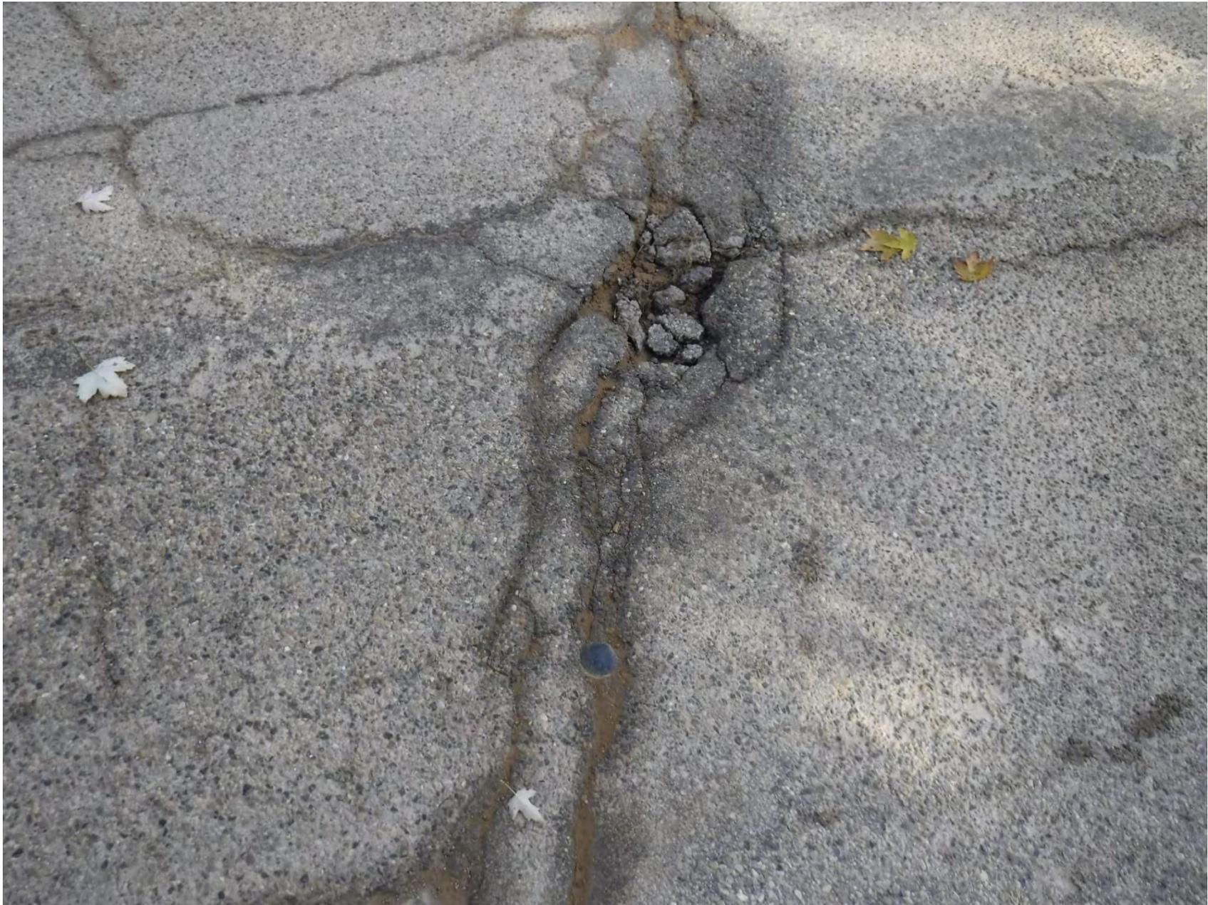
CRACKING WITH SPALL AND EXPOSED DRIFT PIN OVER PIER 2E
