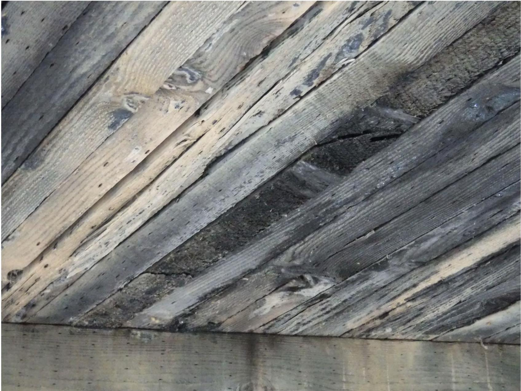
CRACKED DECK BOARD IN SPAN 1E WEST OF SPREADER
