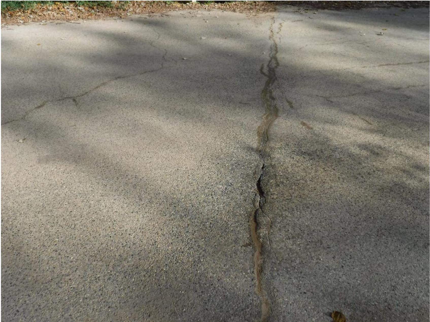
CRACKING AND SETTLEMENT AT WEST REFERENCE LINE
